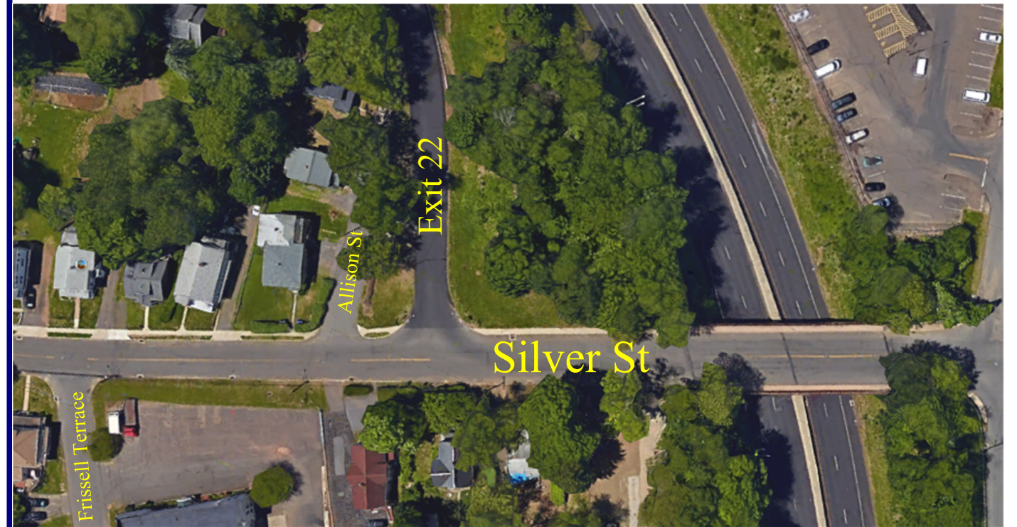
FIGURE 16 — ROUNDABOUT AT EXIT 22 —SILVER STREET INTERCHANGE — EXISTING CONDITIONS
