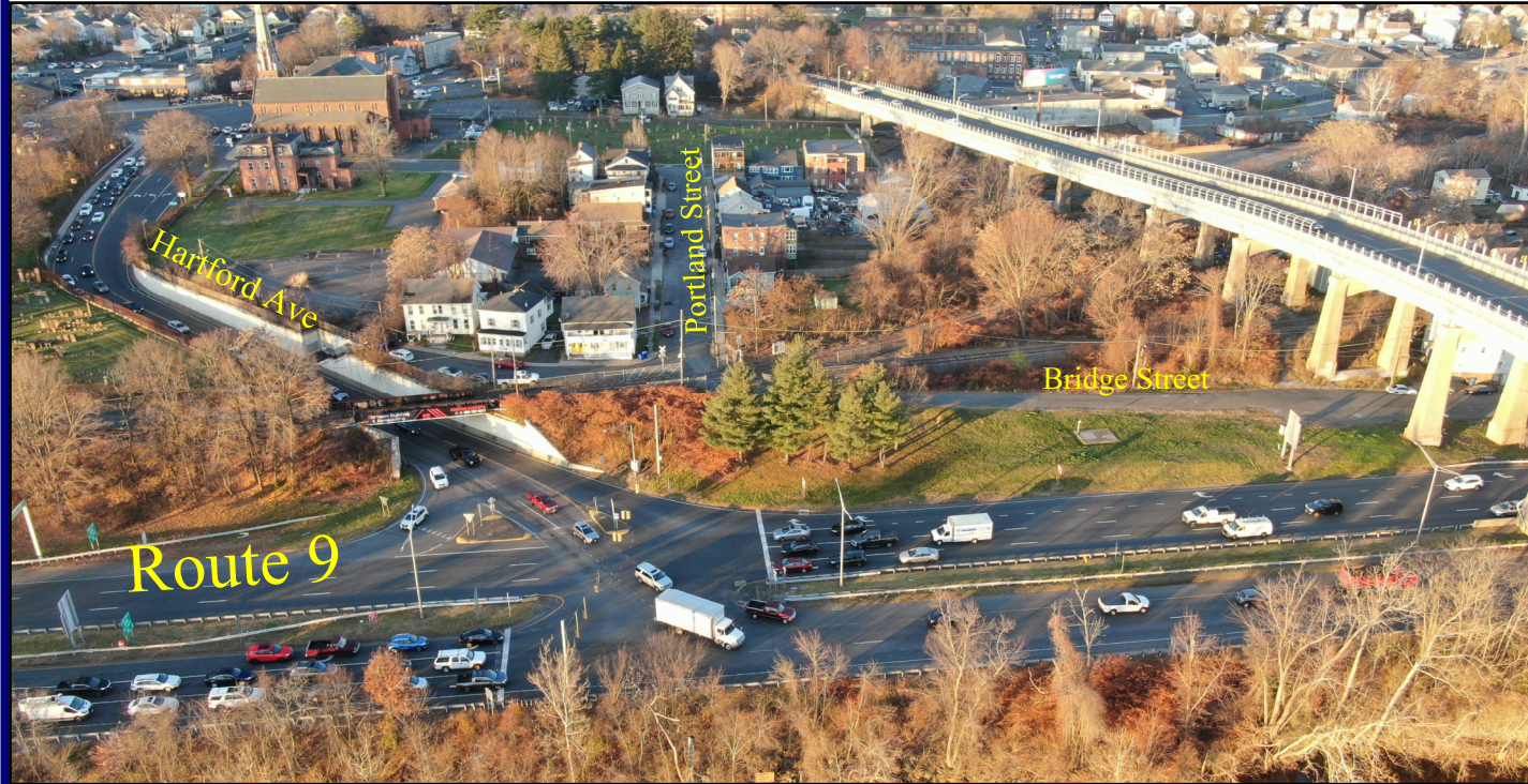
FIGURE 6 — EXIT 24 — ROUTE 9 AT HARTFORD AVENUE — EXISTING CONDITIONS
