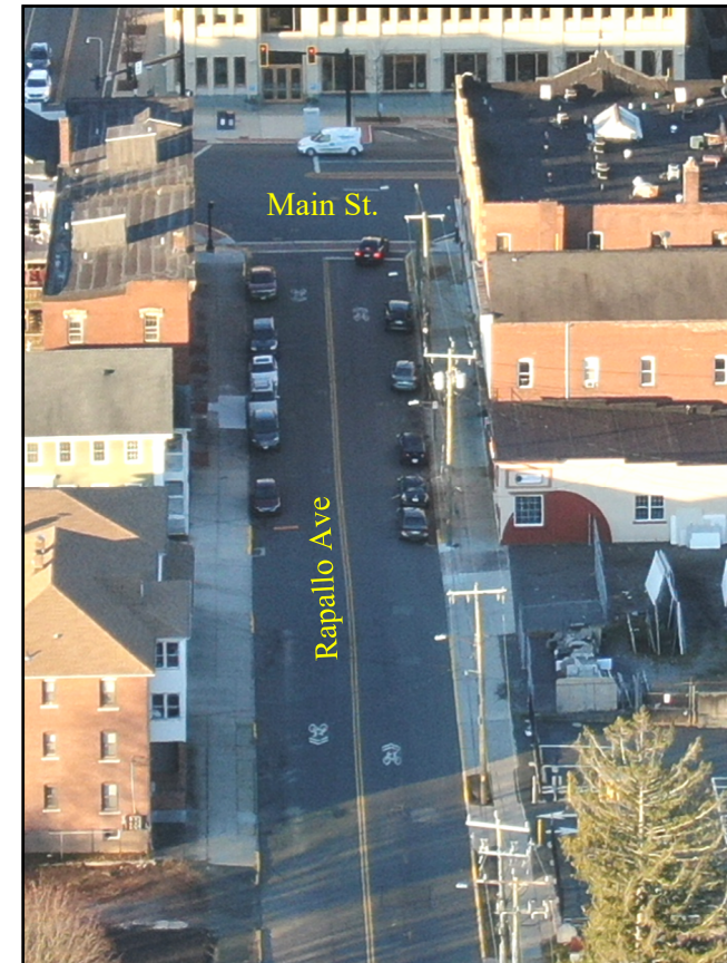
FIGURE 8 — RAPALLO AVE EXISTING CONDITIONS
