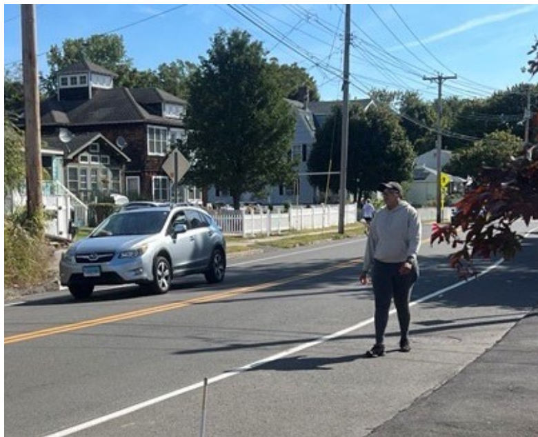
Exhibit 20: Sidewalk at Shell Gas Station (View West)
