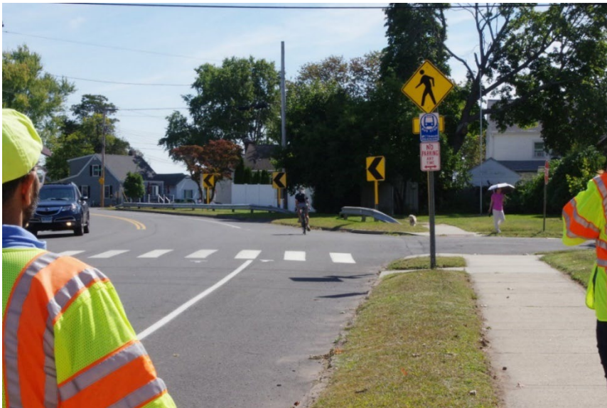
Exhibit 24: Missing Chevron Sign at Morris Street Curve
