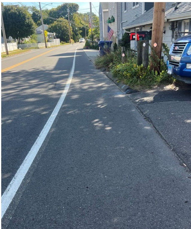
Exhibit 18: Southern Shoulder (View East)
