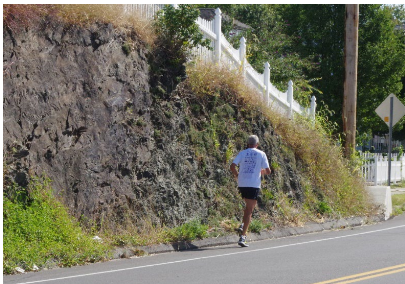
Exhibit 16: Elevated Sidewalk (View East) on South Side of Route 705
