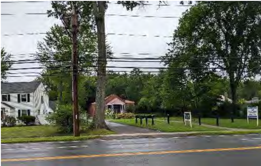
Exhibit 24: Lack of Pedestrian Scale Lighting
