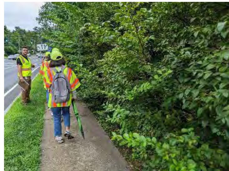
Exhibit 21: Overgrown Vegetation Encroaching Sidewalk
