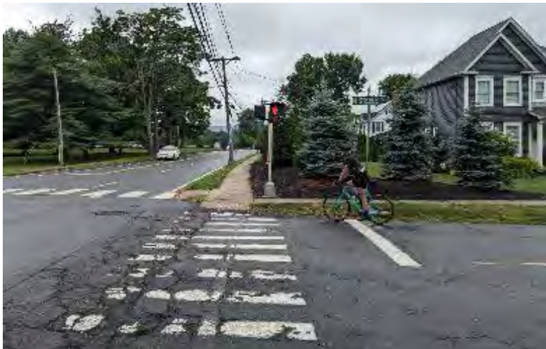
Exhibit 26: Lack of Sidewalk and Narrow Shoulder on South Side of Route 44
