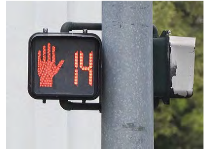
Pedestrian Signal Heads & APS
