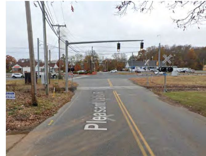
Railroad Crossing Improvements
