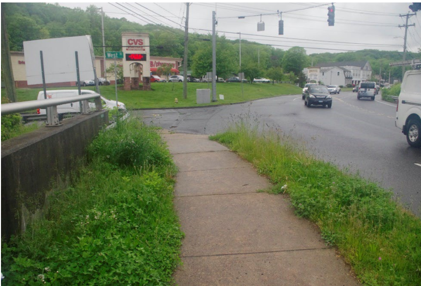
Exhibit 18: Route 67 and West Street Intersection
