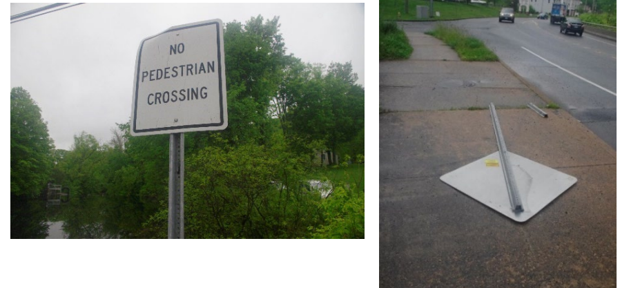
Exhibit 19: No pedestrian crossing sign at West Street intersection and break-away sign damaged near the intersection
