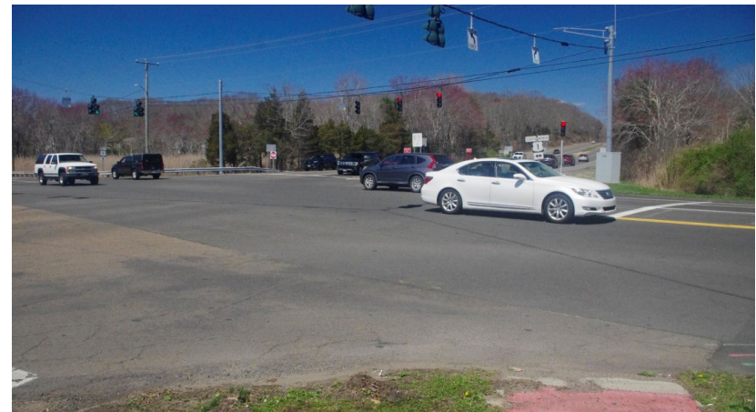
Exhibit 17: Minimal Pedestrian Accommodations at US Route 1 and Hammonasset Connector (Route 450)
