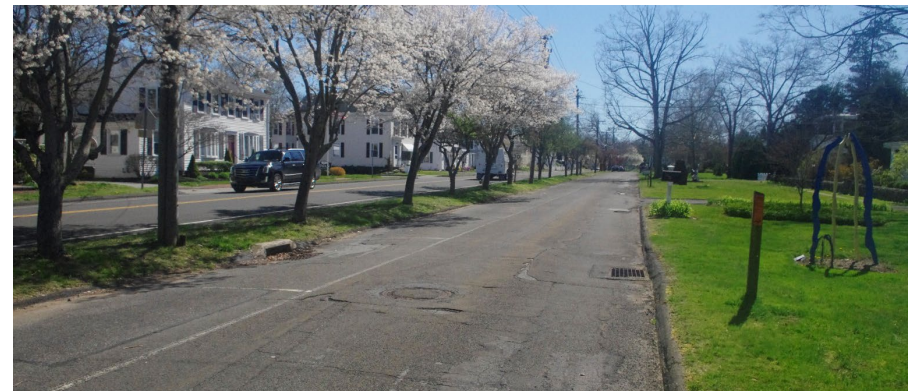
Exhibit 13: Poor Pavement Conditions on Old Boston Post Road
