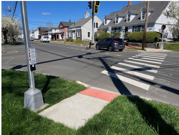
Exhibit 14: Crosswalk Across US Route 1 with Tactile ADA Pad and No Sidewalk
