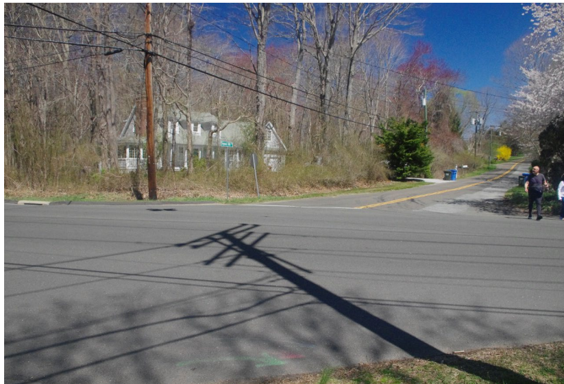
Exhibit 16: No Pedestrian Facilities at Signal Hill Road and US Route 1 Intersection
