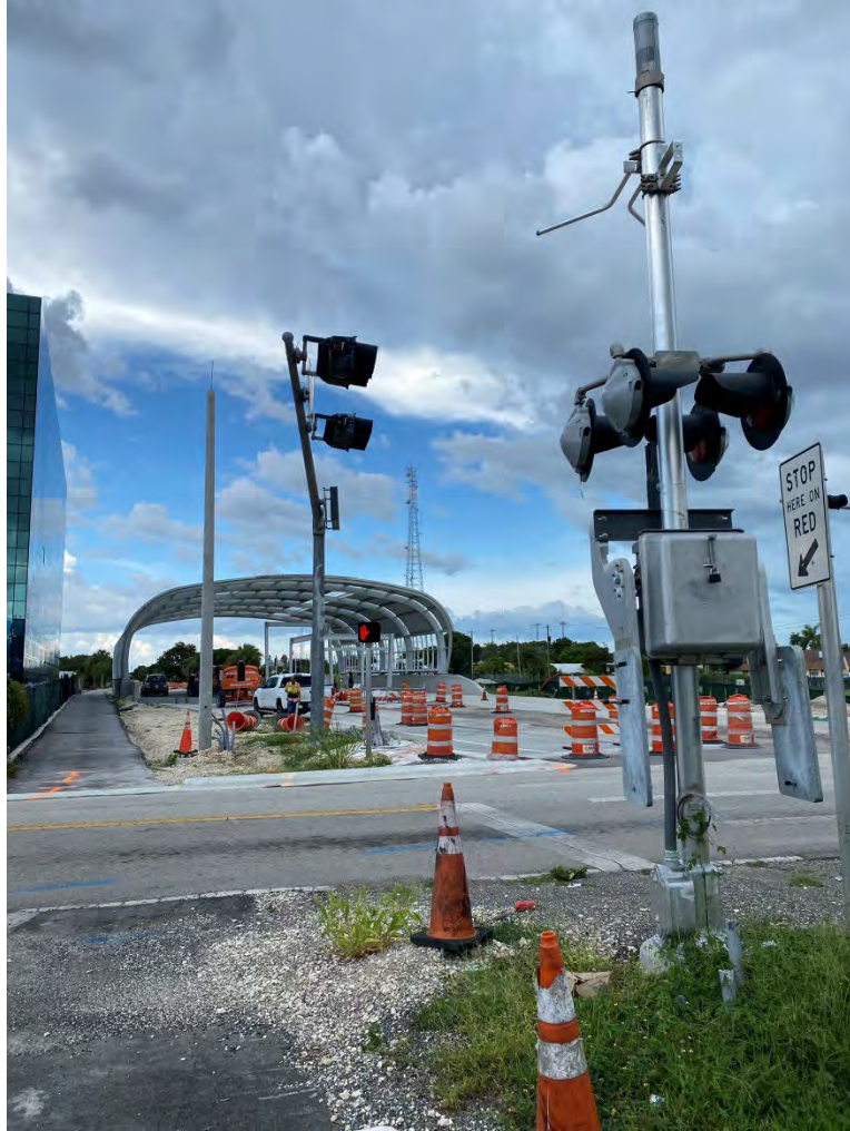
Gates being installed on Miami-Dade Busway ( twitter.com )
