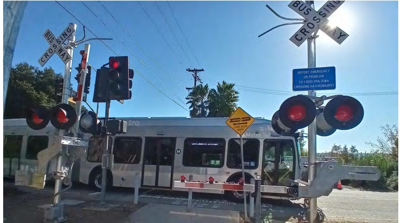
Gates being installed on Los Angeles Pedestrian Crossing ( Youtube.com )
