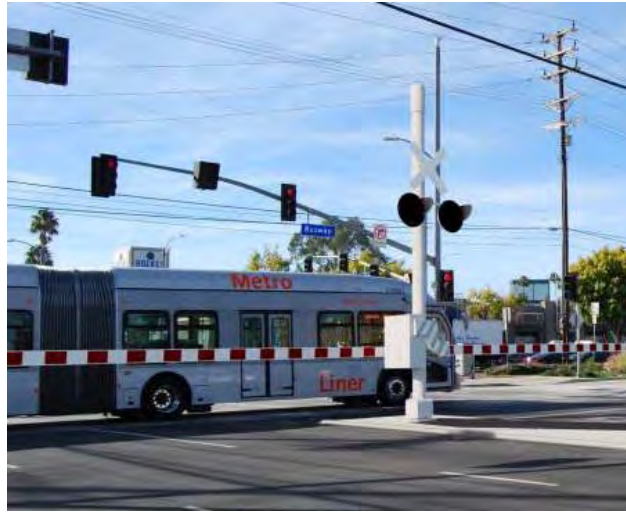
Traffic Gates for Busway Crossings
