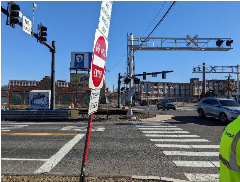
Exhibit 45: Pedestrian signal is blocked by the rail gate
