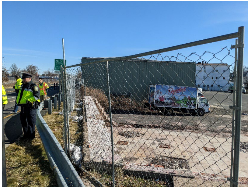
Exhibit 30: Remnants of demolished building at Stanley Street Crossing
