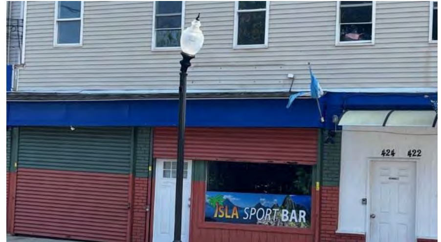
Exhibit 17: Broken Light at on East Side of Route 127 (East Main Street)
