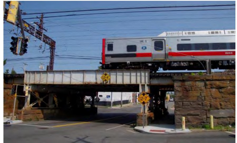
Exhibit 19: Route 127 (East Main Street) Under Rail
