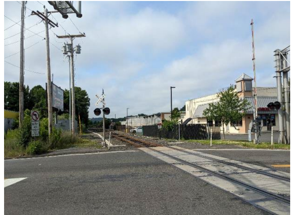
Exhibit 20: Rail Crossing on Division Street
