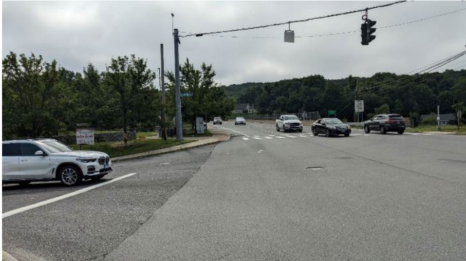
Exhibit 23: Missing Crosswalks on North and South Approaches at Intersection of Division Street and North Division Street
