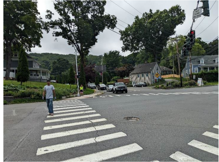
Exhibit 26: Pedestrian Crossings at Division Street/Elm Street and Main Street/Derby Avenue
