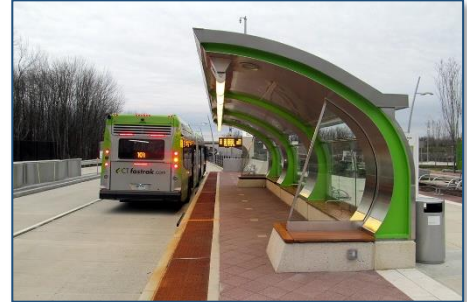
Figure 6: CTfastrak station with curbside tactile warning strips.
