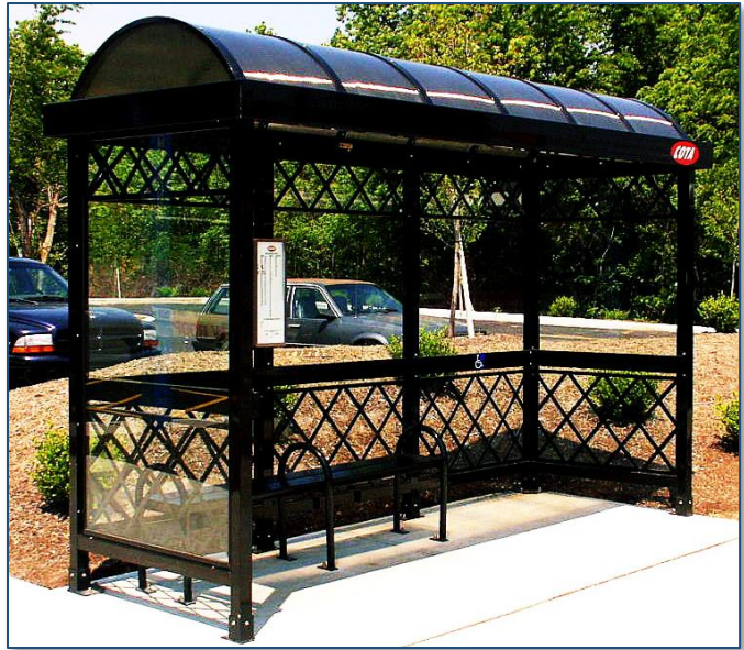
Figure 21: An example of decorative grillwork in a barrel roofed bus shelter.
