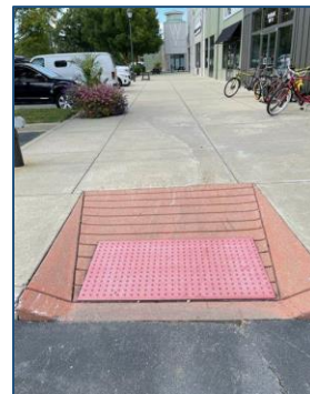
Figure 5: An example of an ADA-Compliant curb ramp at a crossing point.
