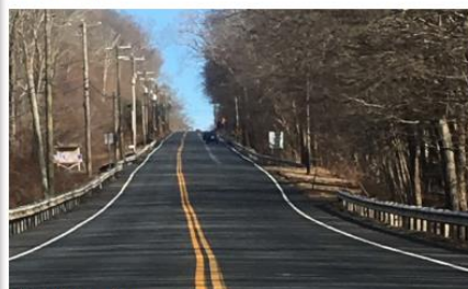
CT-66 Climbing Lanes
