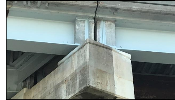
Typical UHPC Beam End Repair
