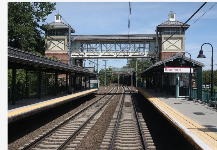
Rail Facilities & Service
