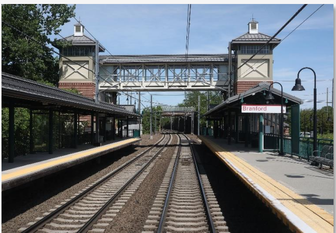
Rail Facilities & Service
