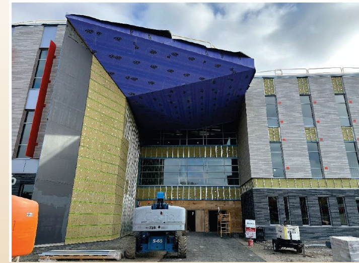
FRONT ENTRANCE CANOPY
