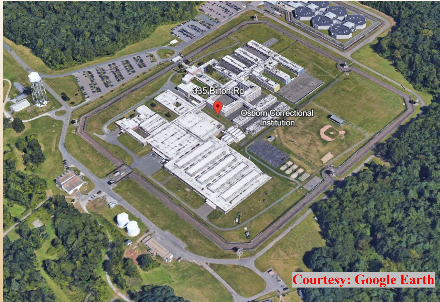
Water Treatment Building at the Osborn Correctional Institution
