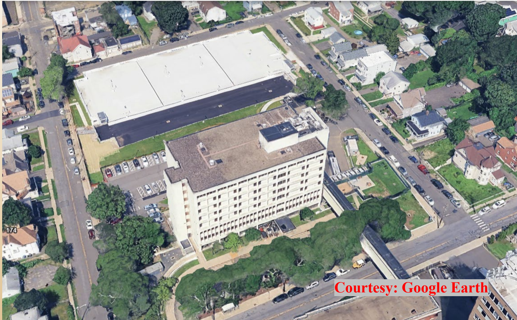
GBCMHC- Sprinkler System and Related Renovations
