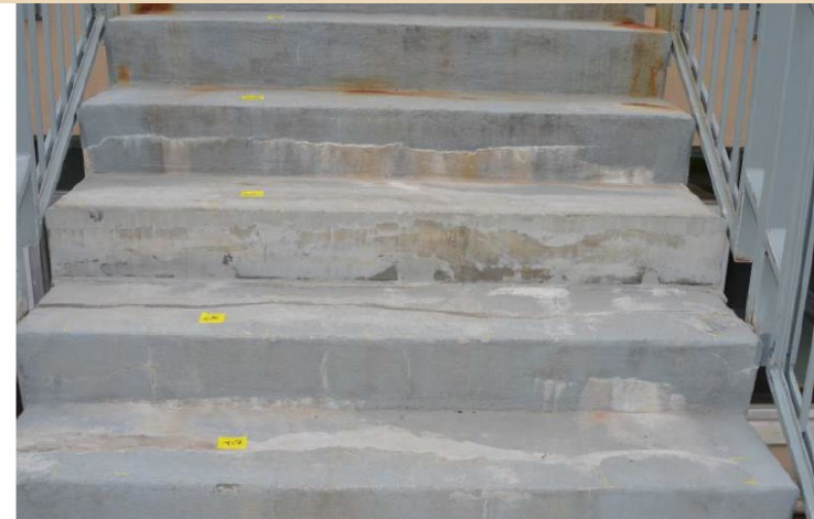
PATCHING AND CRACK FILLING AT STAIRS
