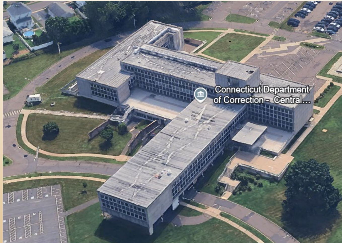
Central Office of Connecticut DOC - Rear Stairs Repair/Replacement
