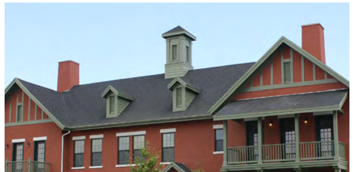
Roof Materials: Asphalt Composite Shingles
