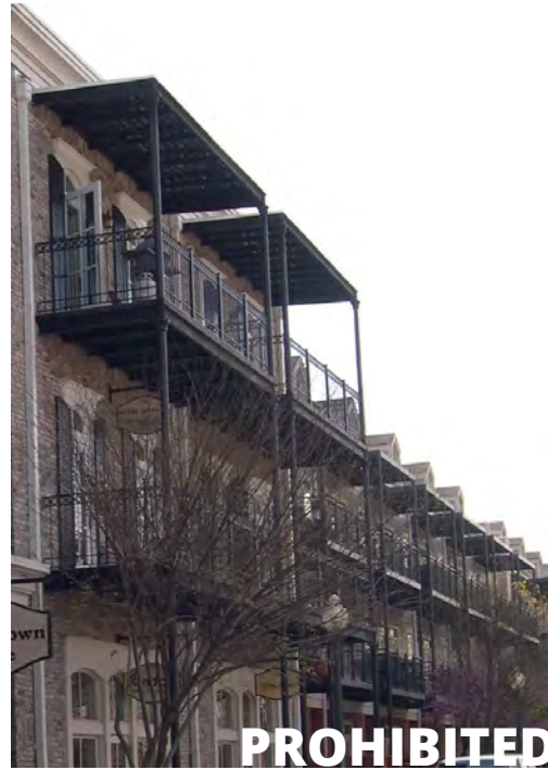
Balconies: Not Permitted
