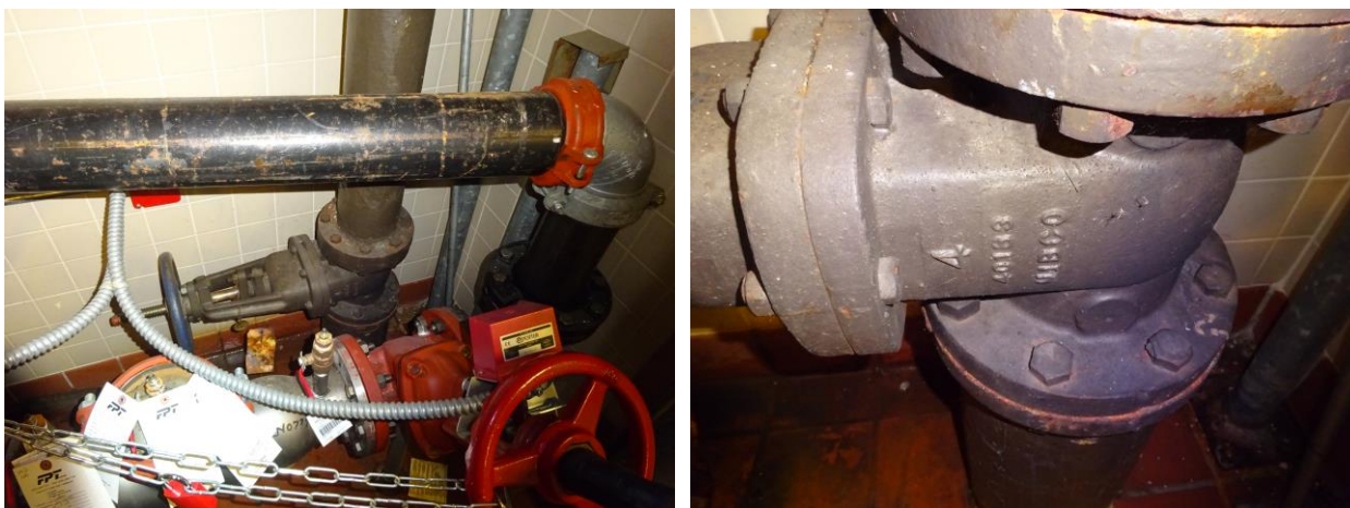
Figure 8: Water service entrance located in northeast corner of middle portion of building.
