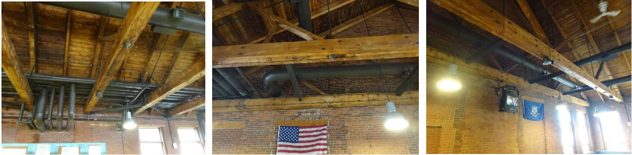
Figure 7: Existing mechanical piping in eastern portion of building (dining).
